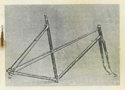
The Modern Design Ladies' Frame, built with Reynolds "531" Tubing, Oscar Egg Lugs and Twin Lateral Stays to give maximum rigidity.
