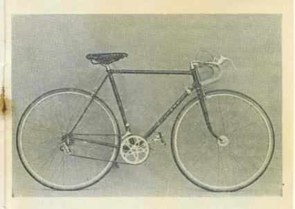
A complete machine suitable for club riding or a spot of racing; built to a price but high-class fittings are used, including G.B. brakes, Brooks saddle, Williams c/set, steel H. P. rims, J. B. tyres.
